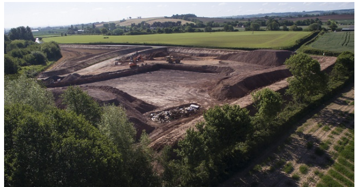
Over 5 acres of land has been excavated at Swang Farm this spring. A notification was accepted for "levelling to ease agricultural use of the field".
